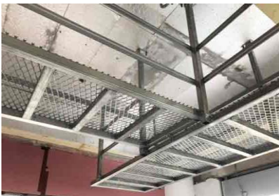
(Additional catwalk have been installed)
